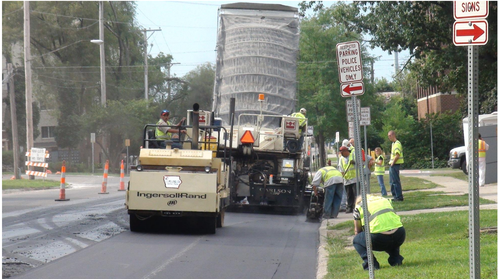
Figure 4.9: Capitol Street job site
