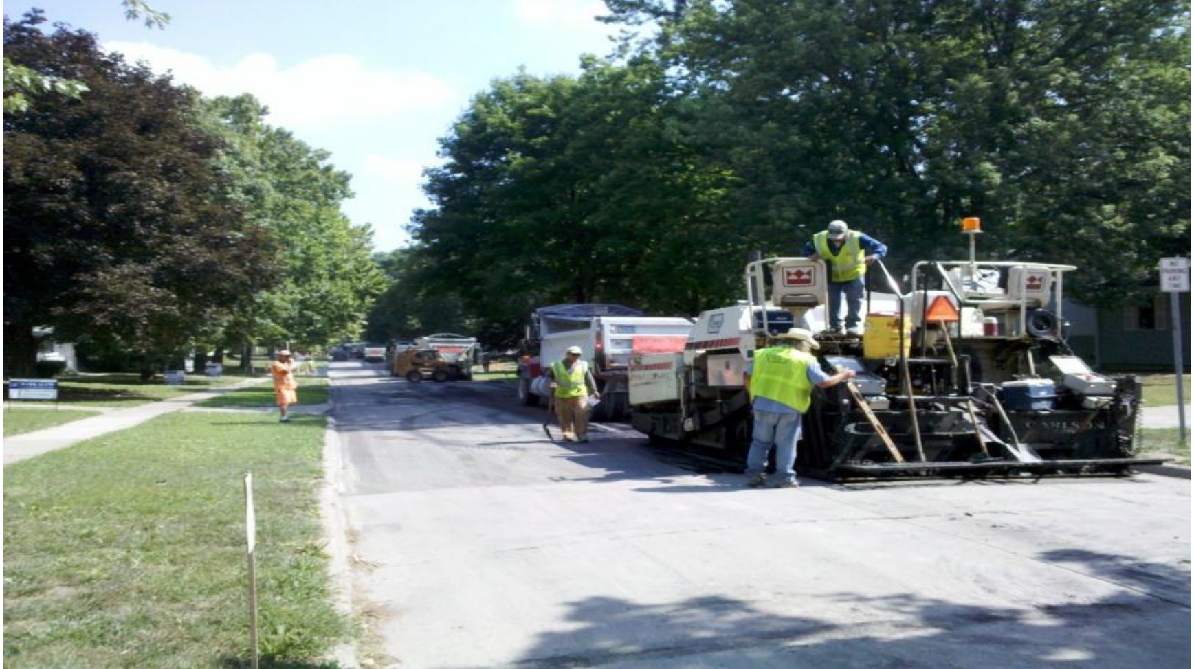
Figure 4.10: Miami Drive job site
